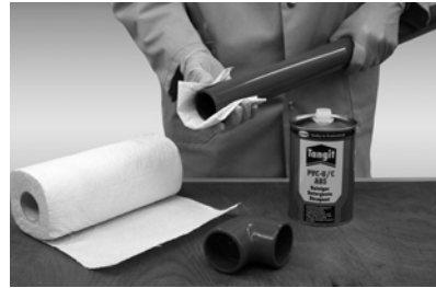
Cleaning the pipe and socket
