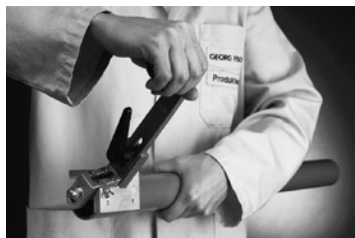
Chamfering the pipe
