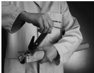
Chamfering the pipe
