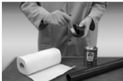
Applying the cement
