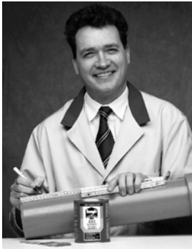
Marking the jointing length
